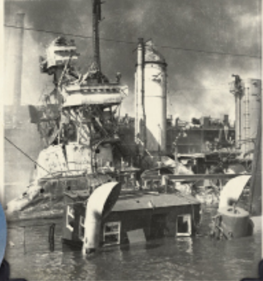
USS SHAW'S bridge was a total loss from fire and explosions.
